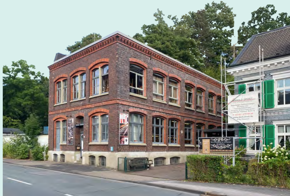
Abb. 39. Bandfabrik Emil Kikuth, 1907
